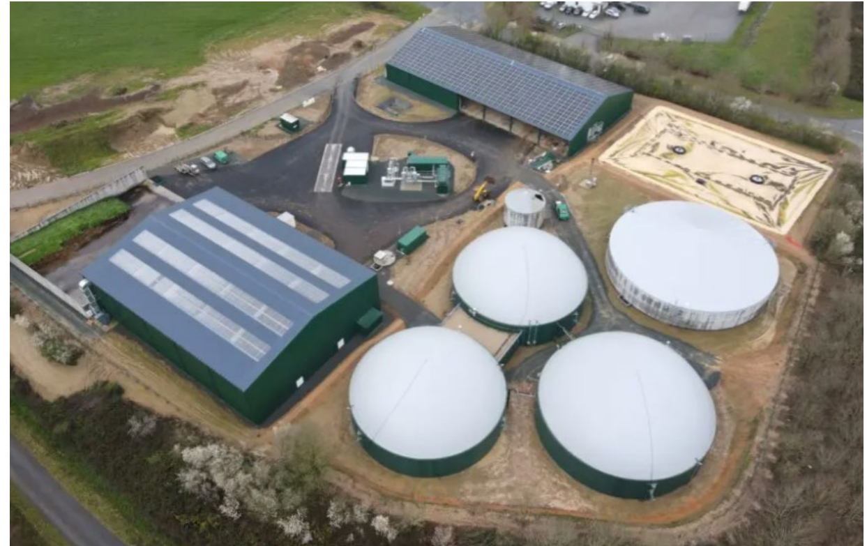
Technique Biogaz (31 000 t/an - 175 Nm 3 /h) – Bournezeau (85)
